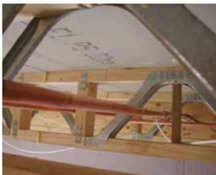
A significant advantage of the **easi-joist®** floor system is the open web design. The space provided by the metal web allows for the easy installation of services within the void.
