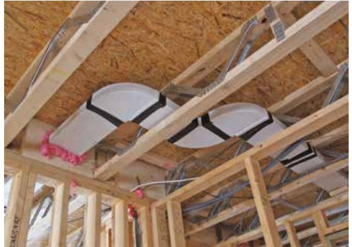
In addition to the need to install traditional ventilation services in bathrooms and kitchens, Government initiatives for air tightness may require the installation of mechanical systems for heat recovery and air exchange. The open web design provides an ideal zone for the passage of ducting for these devices.
