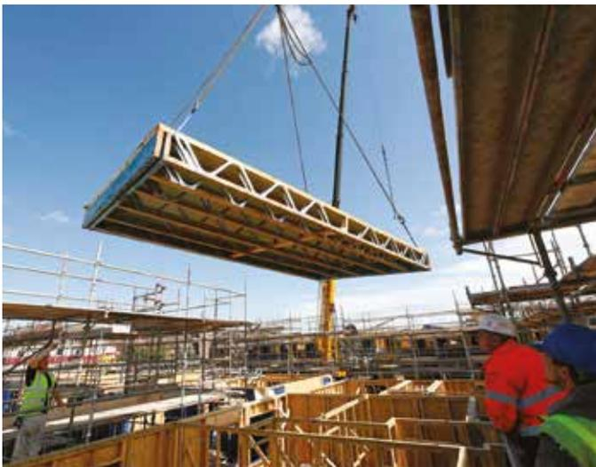
**easi-joist®** is ideally suited for the manufacture of floor cassettes. Along with the advantages on-site for the accommodation of services and long-term stability, the wide bearing surface makes it easier to lay out the joists in preparation for adding rimboard, blocking and decking during assembly of the floor cassette.
